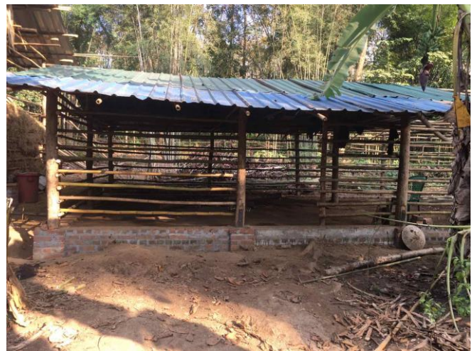
Completed cow barn.
