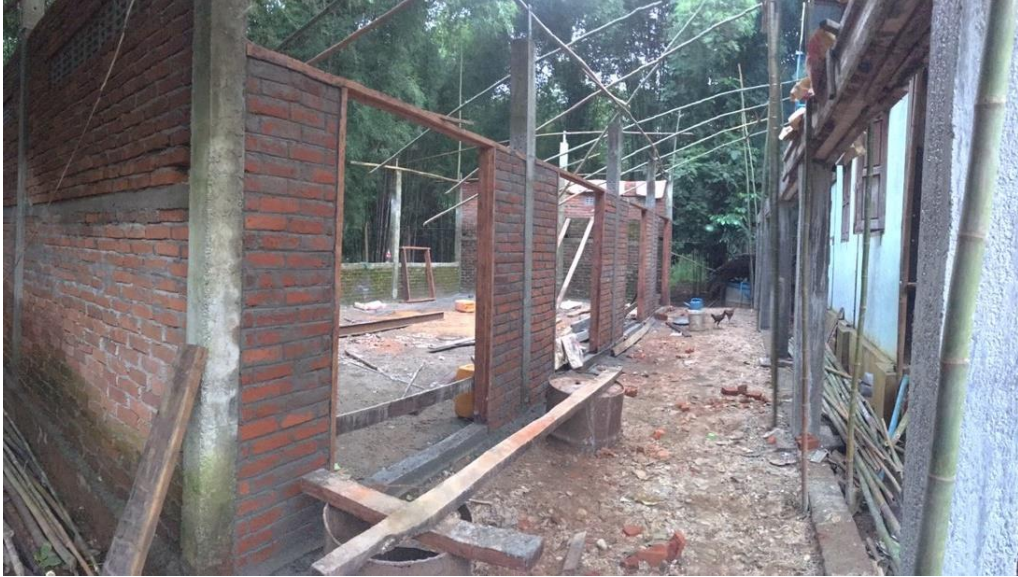
Ground floor with most bricks already in place
