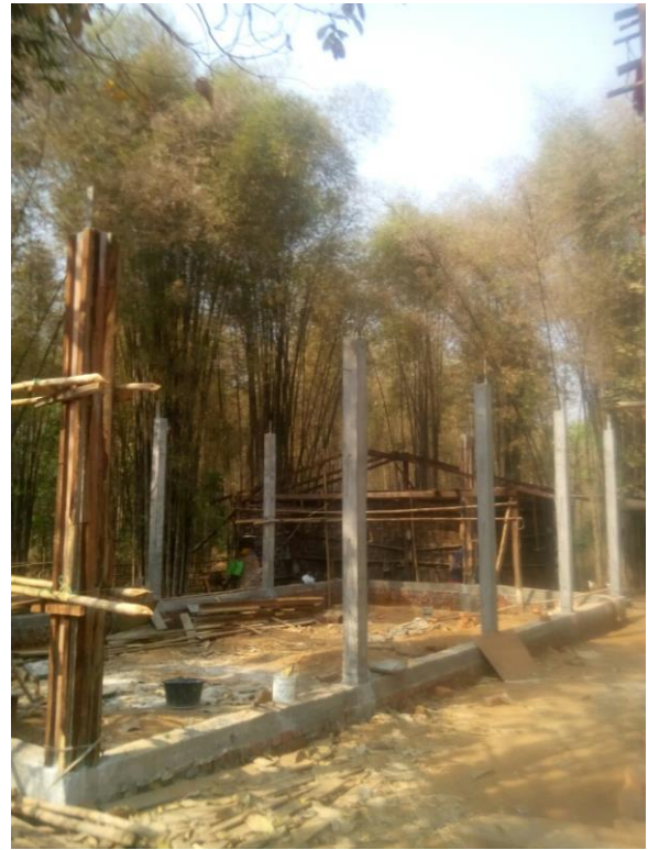
Foundation with posts for the eating area
